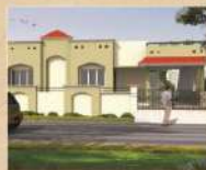
POWER CITY PHASE II
